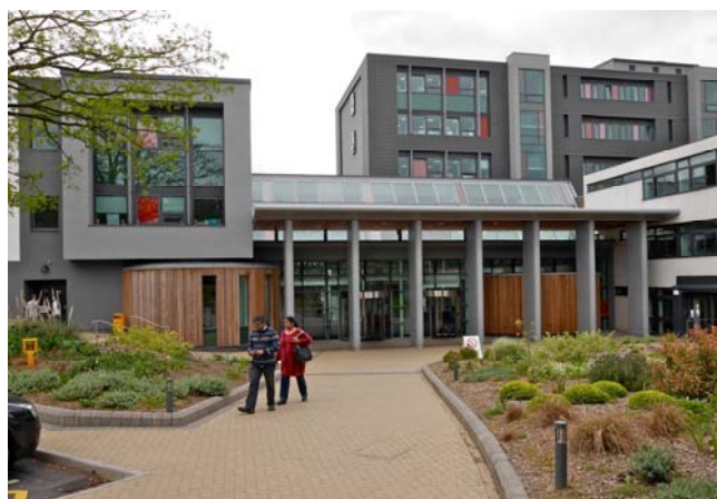
New foyer at Warwickshire College
